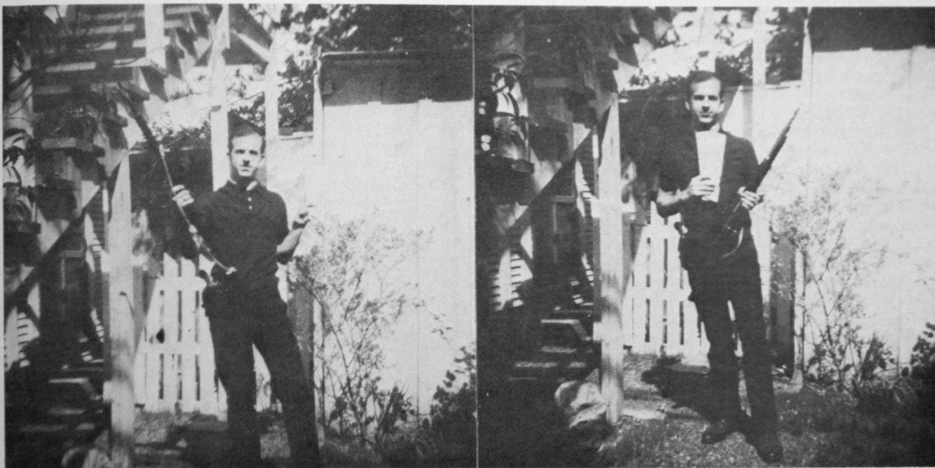
Figure 12. The camera was level for the view on the left, as evidenced by the parallel vertical lines in the background. The camera was tilted down slightly for the view on the right, placing the head farther off the lens axis which resulted in elongation due to the wide-angle effect.
